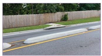
Figure 4: Median breaks allow stormwater to drain while reducing water volicity
